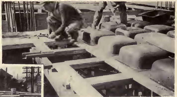
ON THE LEFT FORMS IN PLACE READY TO RECEIVE DOMES
